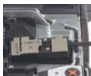
Drop cable splicing with fiber holder system
